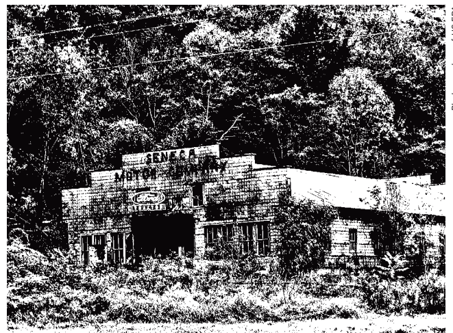
Photo courtesy of US EPA
