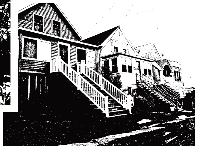
Photo courtesy of US EPA
